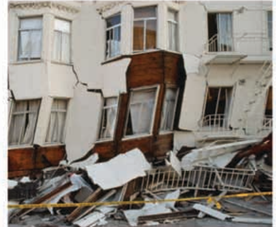
On October 17, 1989, San Francisco experienced a large magnitude (7.1) earthquake.
