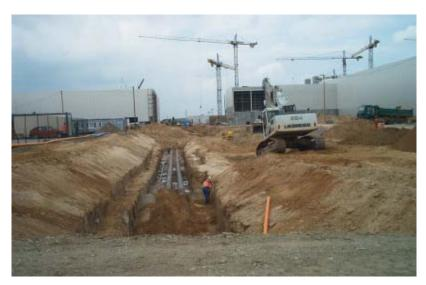
Photo 6: Parallel connecting pipeline to a sprinkler sub-central room
