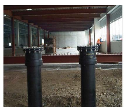
Photo 8: Prepared connection to the sprinkler sub-central room
