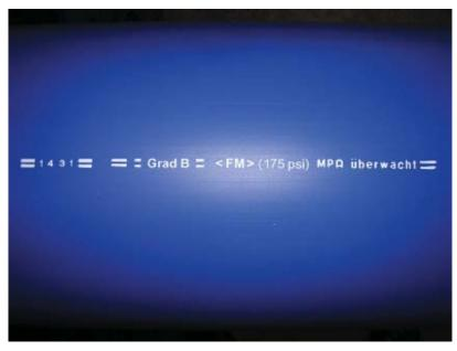
Photo 5: Marking in accordance with FM standard 1610
