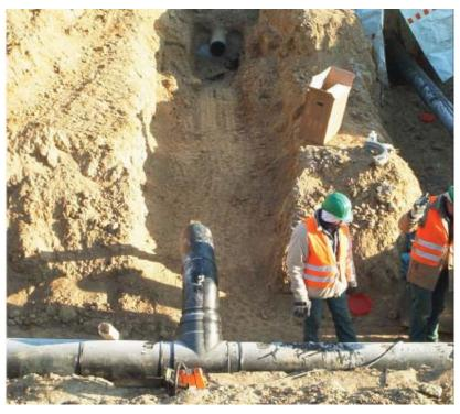
Photo 7: Branch from the main pipeline (DN 300) to the sprinkler sub-central room (DN 250)
