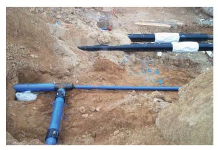
Photo 2: Agruair compressed air pipe and fire main (background)
